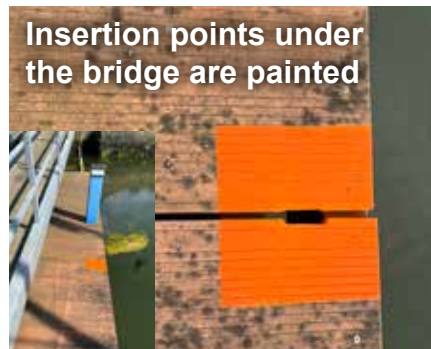
Push bracket between boards
